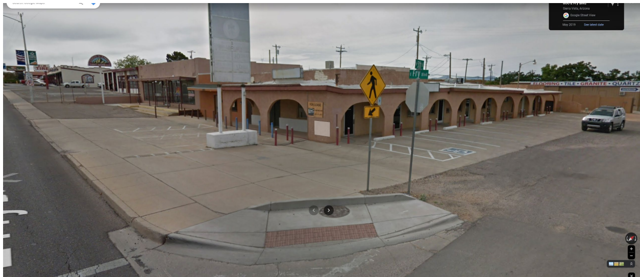
Subject Property-597 E. Fry Blvd. Looking northwest from Fry Blvd.
