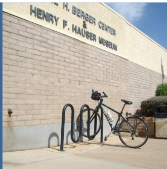
Rack too close to the wall and the front wheel can easily be removed resulting in stolen bike.
