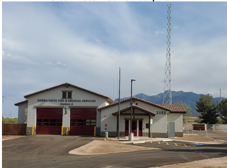
Site Photo – June 16th, 2022
