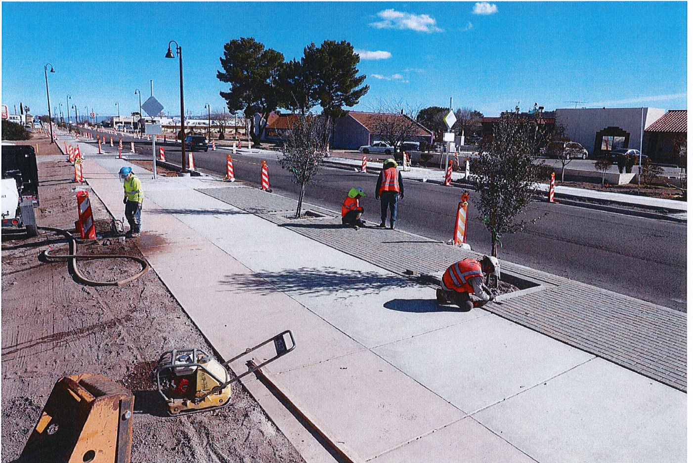
PHASE 1 CONSTRUCTION – W FRY
