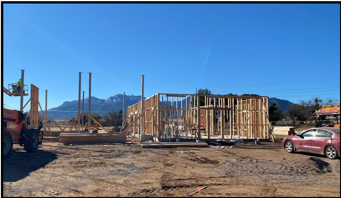
Site Photo – Jan 6, 2022
