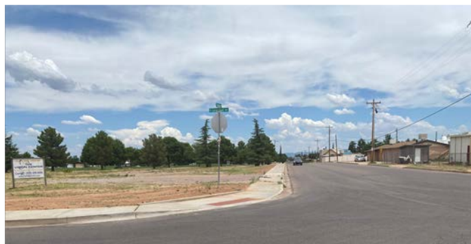
ADA Ramp/Sidewalk - Theater Dr./Carmichael Ave.
