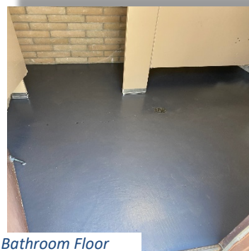
New Stone Bathroom Floor
