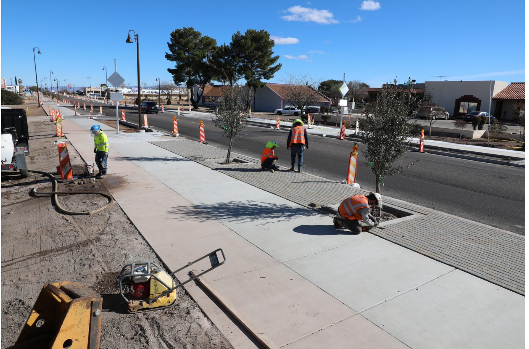
PHASE 1 CONSTRUCTION – W FRY
