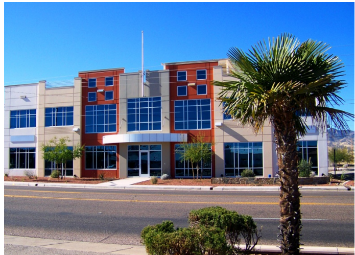
Building, North Garden Avenue
