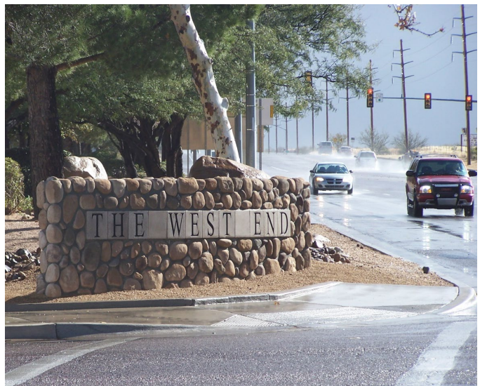
West End entryway monument walls
