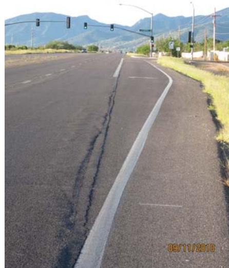
SR 92 and St Andrews Drive, looking south – bicyclists do not have a designated area while waiting to proceed through the intersection
