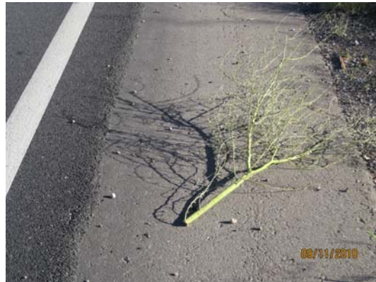
Example of debris on SR 92 Photo Source: Thomas Armstrong
