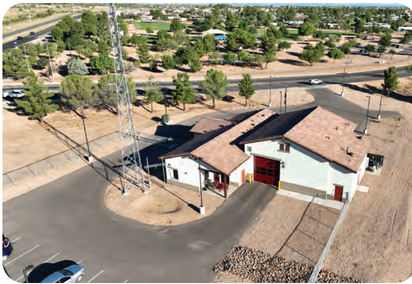
Aerial view of SV Fire Station #4 (EMS Substation)
