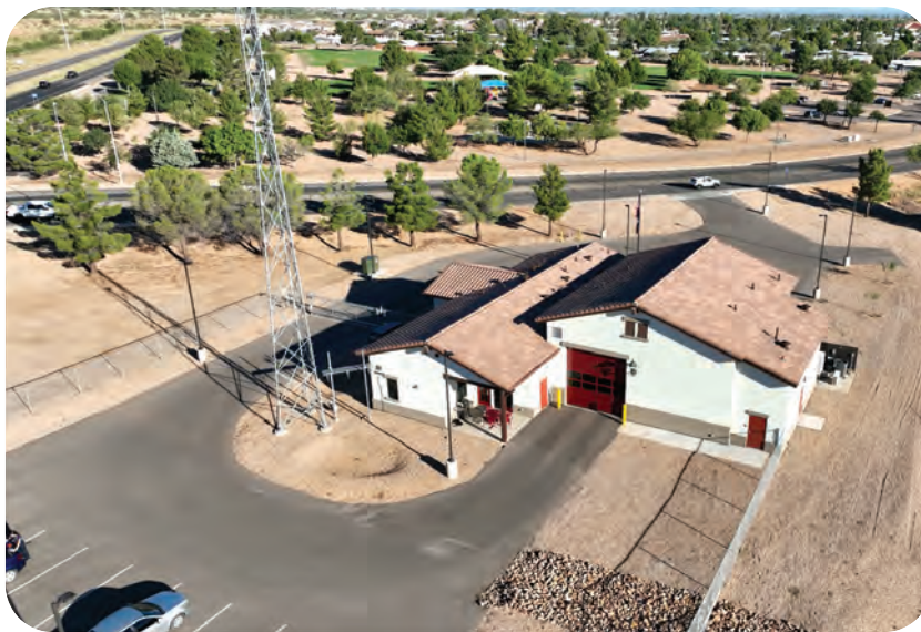
Aerial view of SV Fire Station #4 (EMS Substation)
