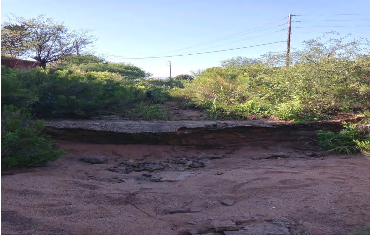
Figure 4.8.5 – Grade Control along the 3rd Street Drainageway about 1000-feet Downstream of Fry Blvd.
