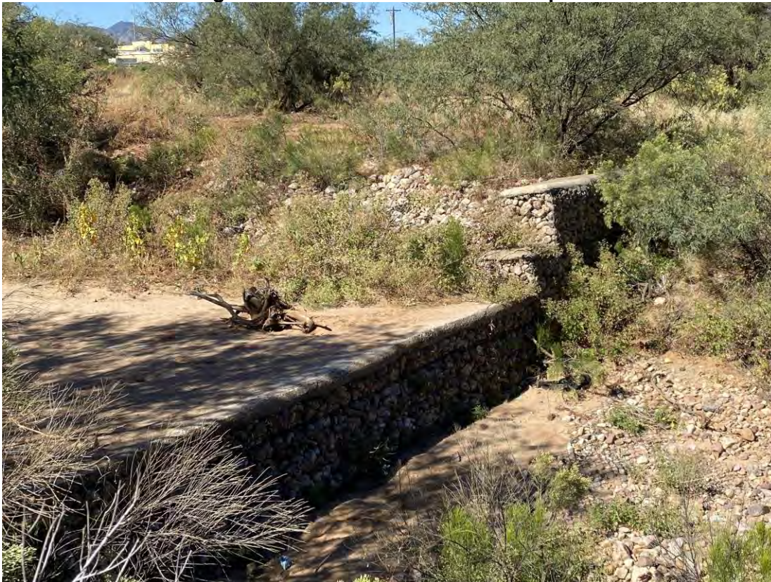
FIGURE 9.29 - Existing Grade Control Structure 140-ft Upstream of SR-90
