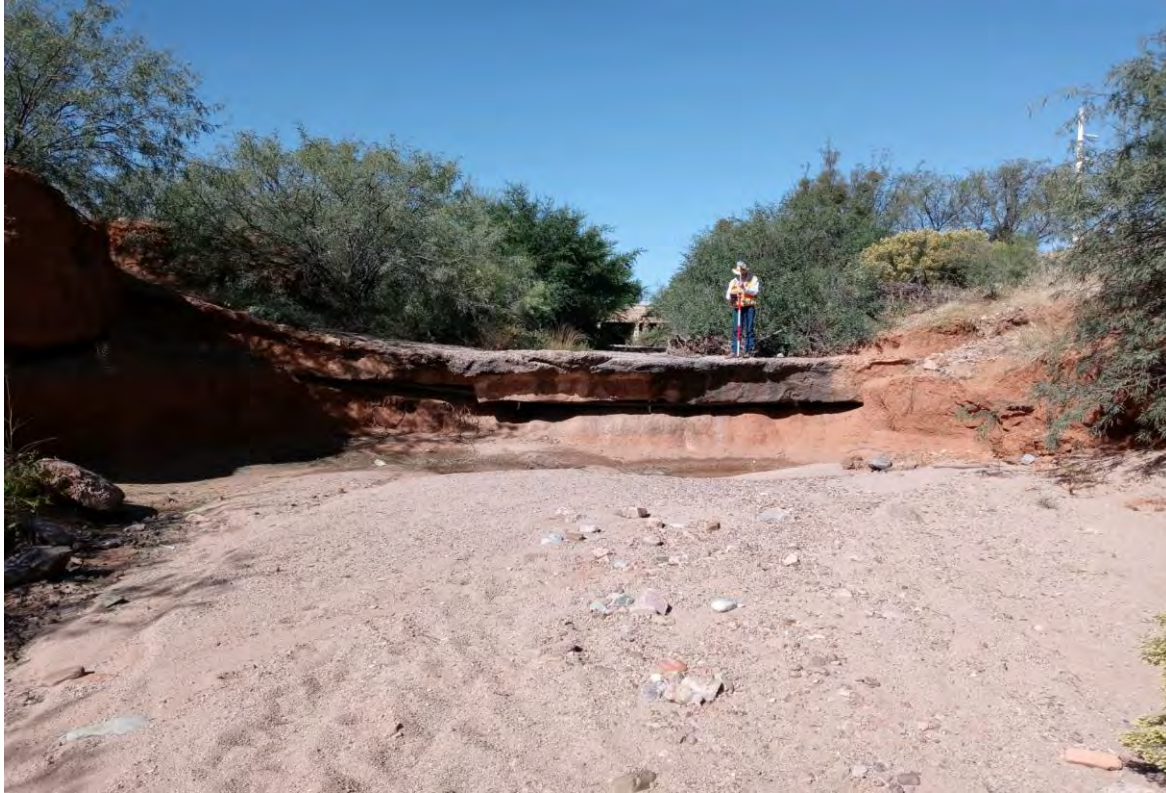
Figure 9.22 - Existing Grade Control 200-ft Downstream of Coronado Dr
