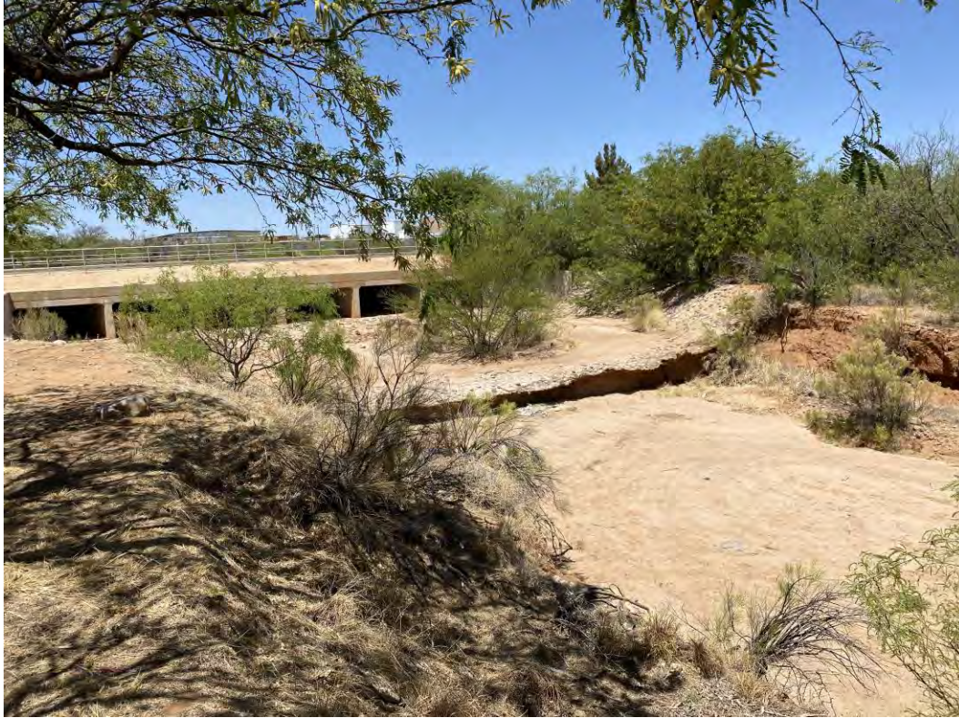
FIGURE 9.18 - Colombo Avenue Culvert Outlet
