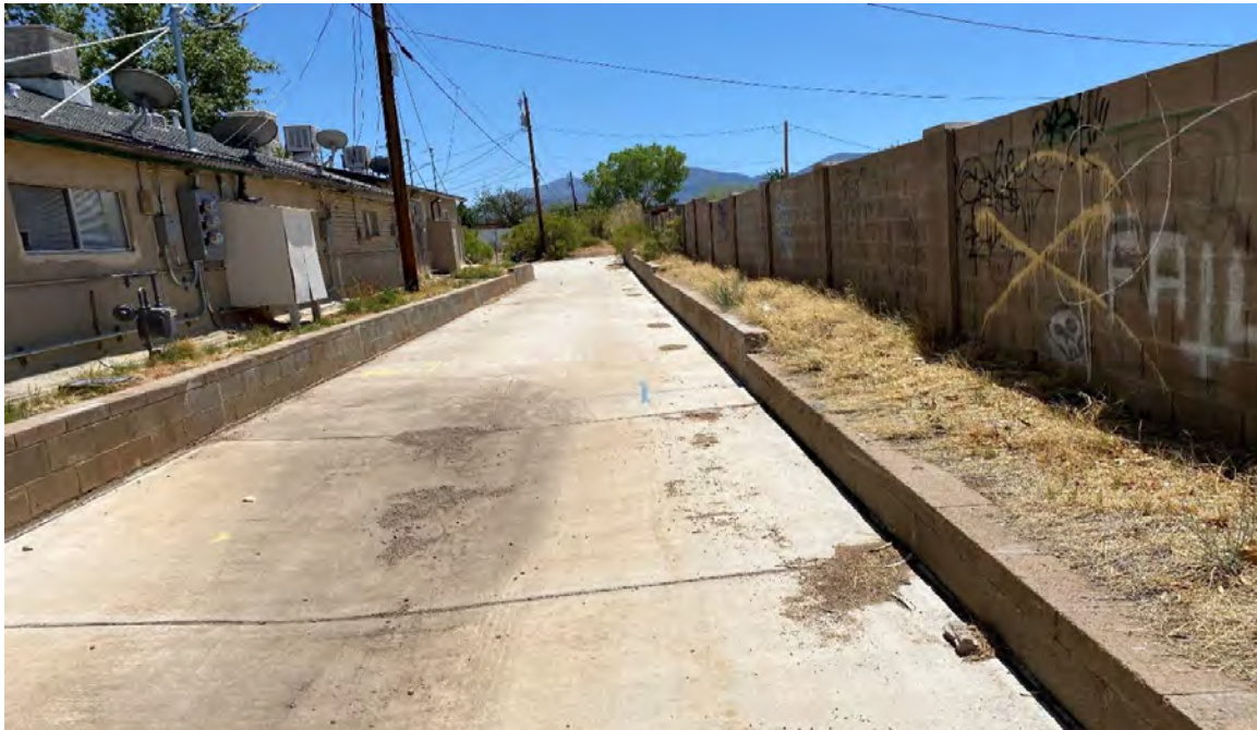
Figure 9.4 - Channel Connecting Fab Ave Drainageway to 66-inch Storm Drain Inlet
