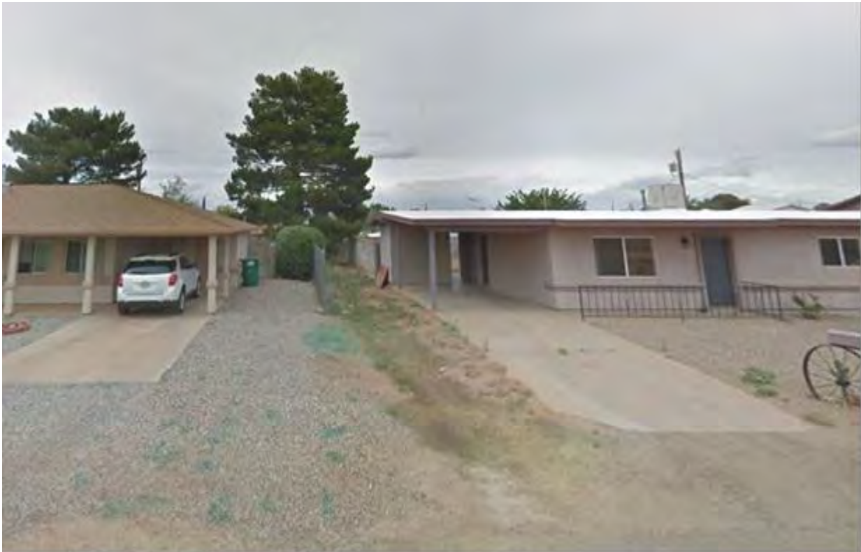
Figure 4.1.2 - Timothy Ln –Sulger Subdivision Drainage Swale between Residential Lots
