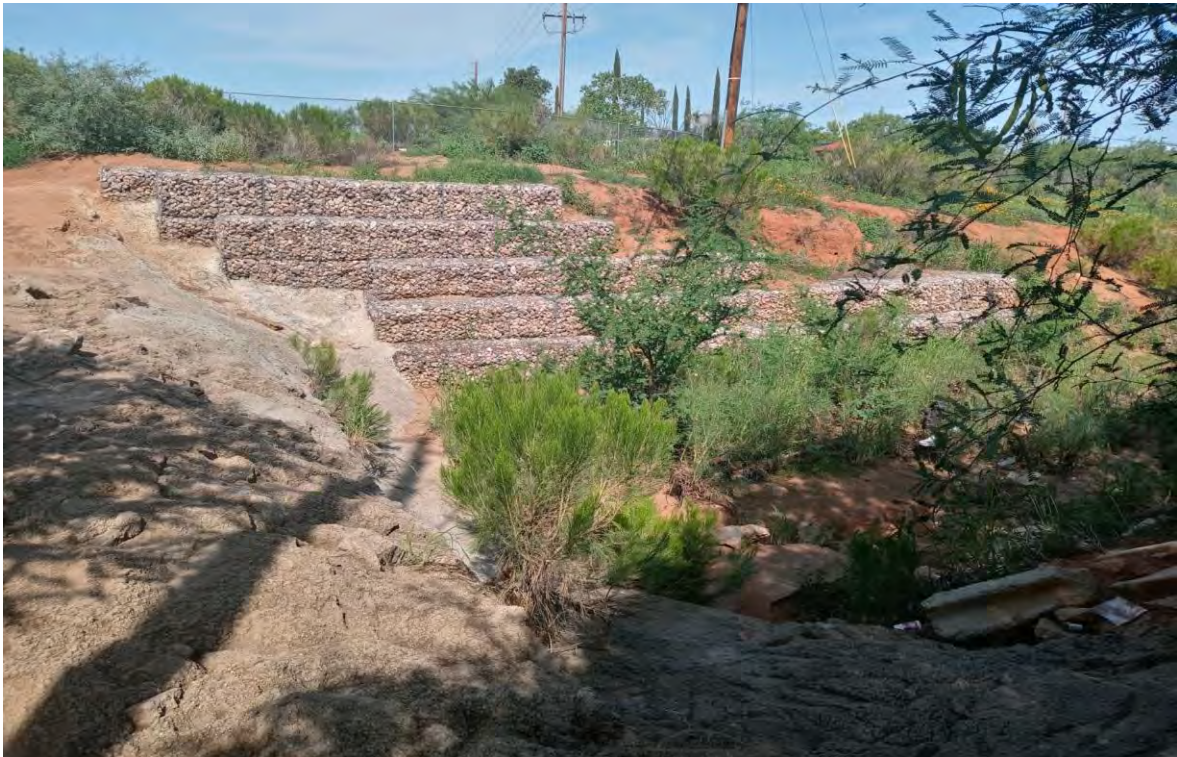
Figure 4.8.6 - 3 rd Street Drainageway about 560-feet Downstream of Fry Blvd.
