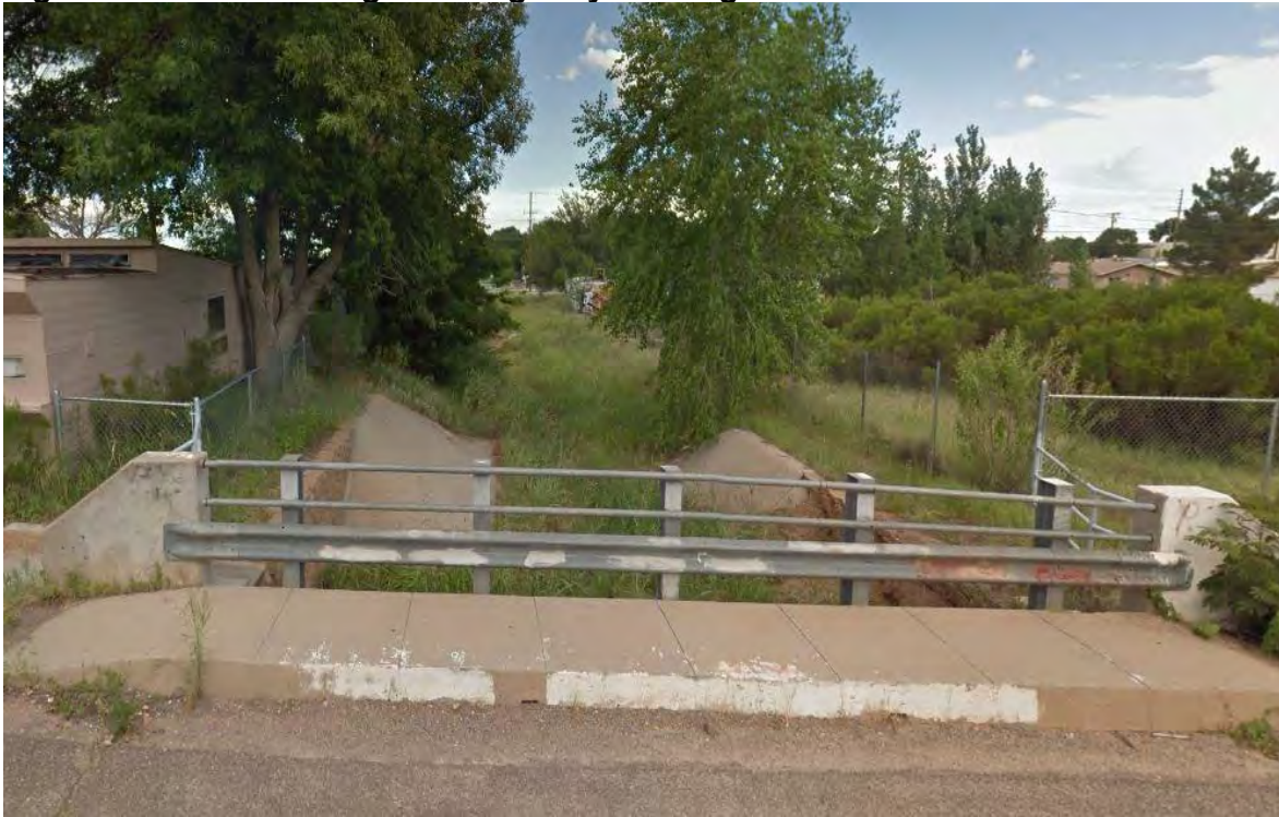
Figure 4.2.5 - Vista Village Drainageway Looking Downstream from 6th Street
