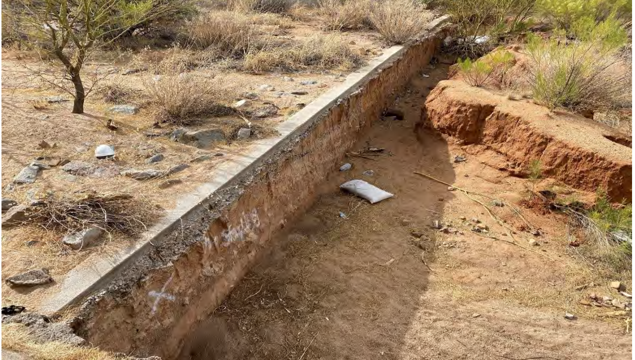
Figure 4.4.1 - Kings Manor Wash Grade Control at Savannah Springs Apartments
