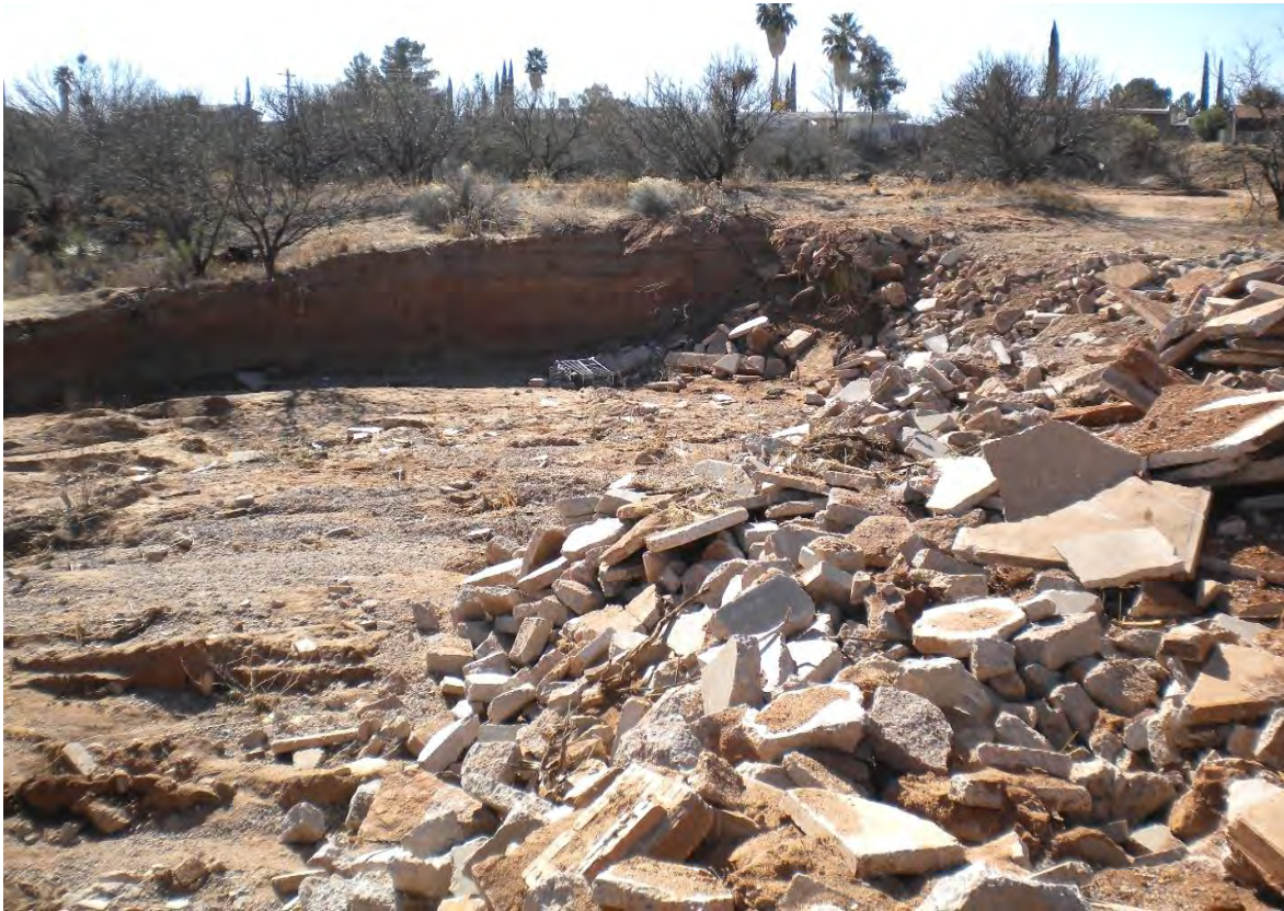
Figure 5.1.1 - Headcut along Coyote Wash Downstream of Foothills Drive
